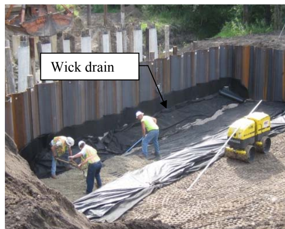
a.) Engineering fabric placement
