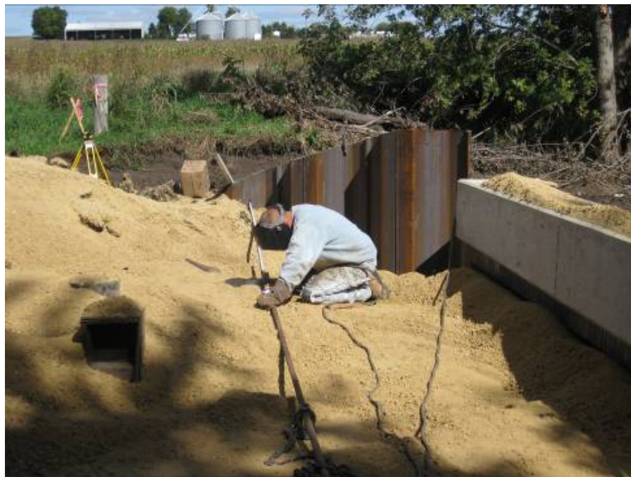
Figure 5-20. Installation of wingwall tie.
