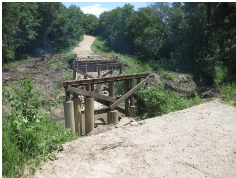
b.) Superstructure removed
