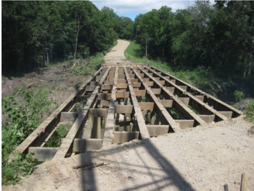
a.) Timber decking removed (exposing steel girders)
