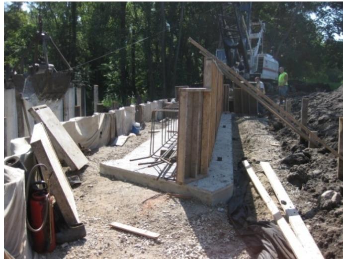
Figure 5-83. Reinforced concrete spread footing on west abutment.
