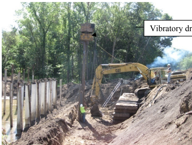
a.) Vibratory pile driving
