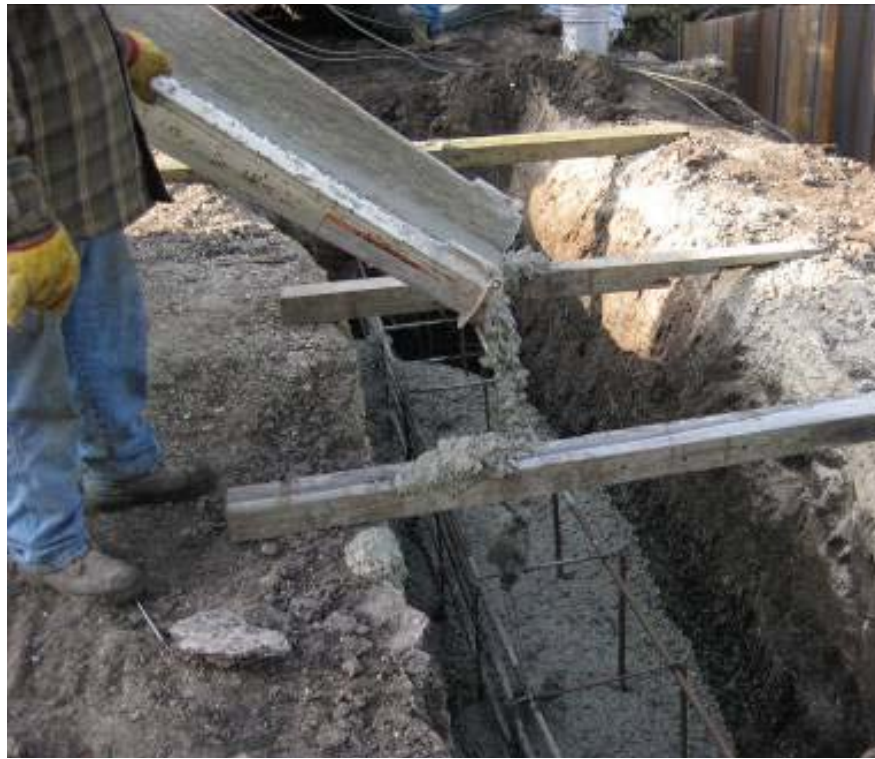
Figure 5-19. Reinforced concrete deadman placement behind east abutment.
