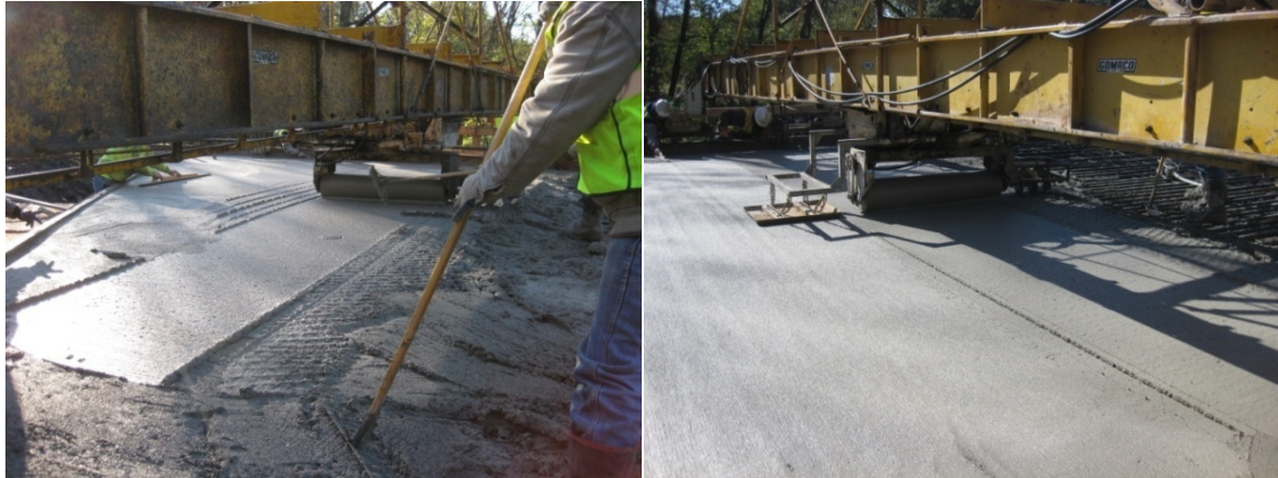
a.) Unfinished concrete after placement
