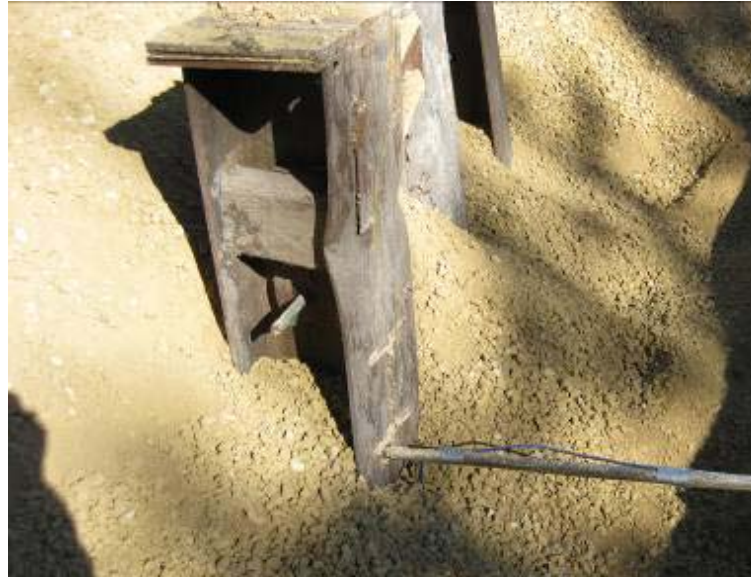
Figure 5-21. Tie rod to H-pile connection.
