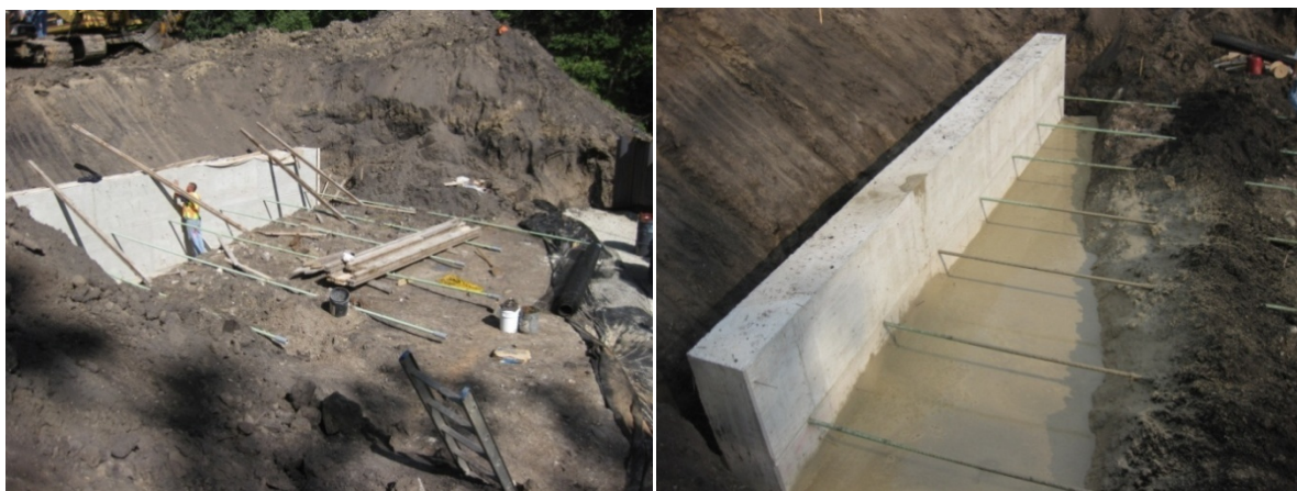
Figure 5-74. Reinforcement placement for concrete deadman.
