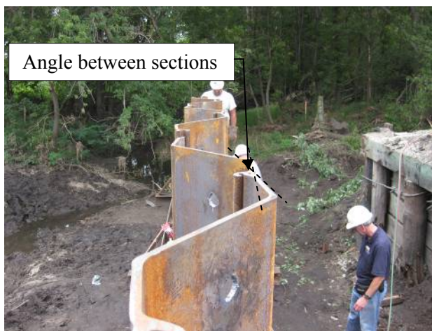
a.) Angle between sections
