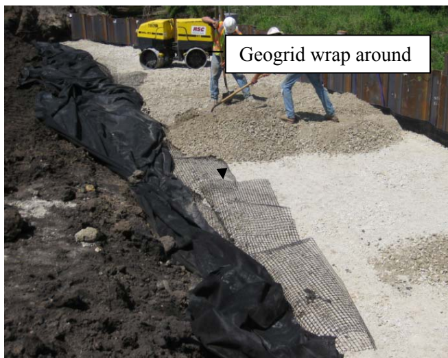
a.) View of geogrid wrapping around layer of backfill
