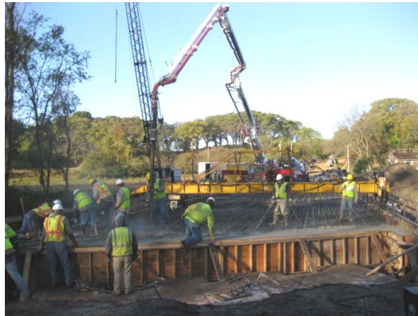
Figure 5-89. Concrete pumping for continuous concrete slab.
