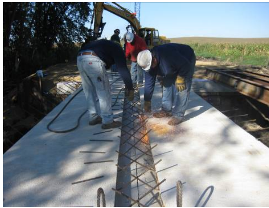
Figure 5-31. Finishing of bridge deck joints.
