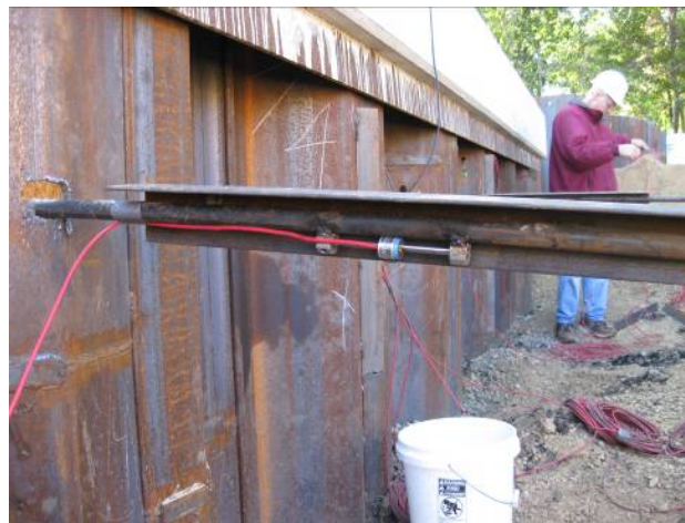
Figure 5-23. Tie rod strain gage installation.
