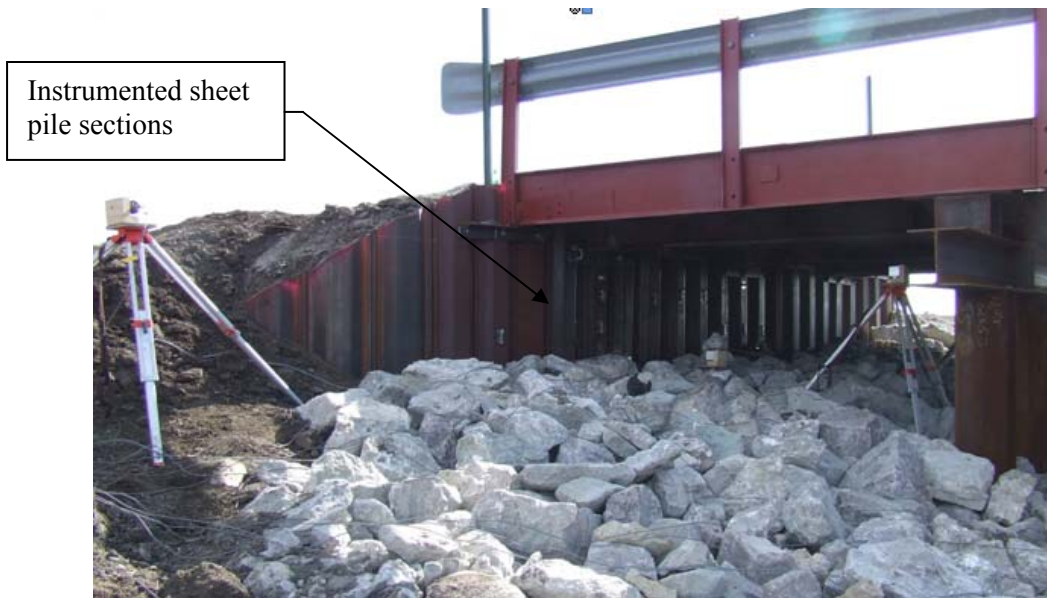
a.) View of abutment and pier
