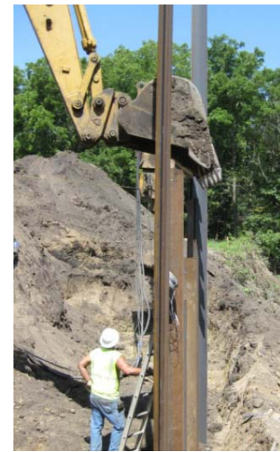
b.) Initially set and held with excavator boom
