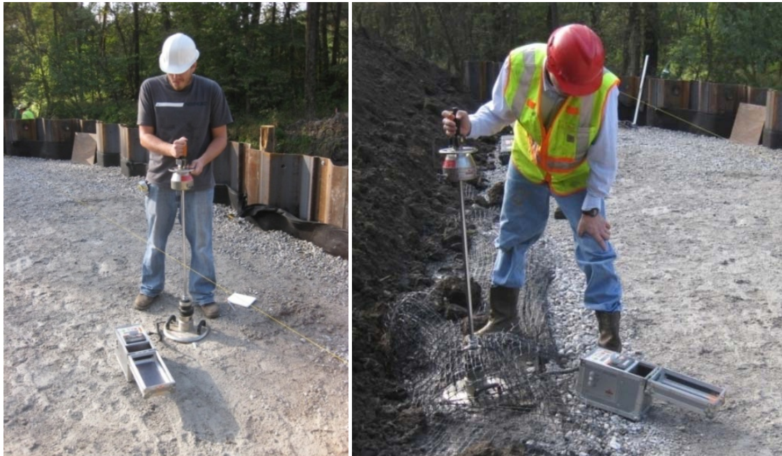
a.) Testing on abutment backfill at base of spread footing
