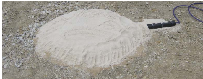
a.) Fine silica sand bedding for earth pressure cell
