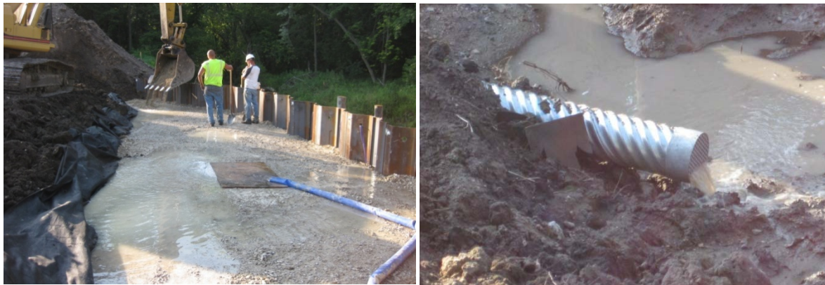
a.) Pumping water from stream
